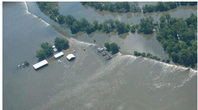
Flooding over levee banks
